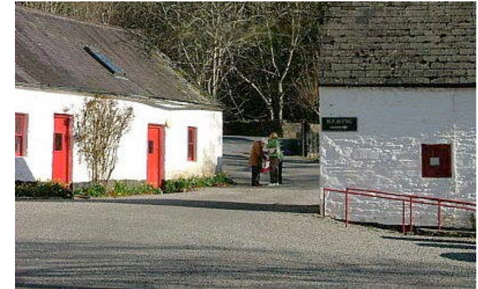
Left, and far left: Traditional farm and fields and Ward River boundary are an opportunity to conserve the farm as an active museum of country life in Fingal with agricultural artefacts and, traditional furnishing of the cottage. The outbuildings might be used as a shop, much in the way the Avoca Hand weavers have retained their traditional buildings in Avoca village. Within the village, it is an attractive opportunity to incorporate an active recreational and educational purpose with county wide interest as a sustainable conservation project for both buildings and landscape.
