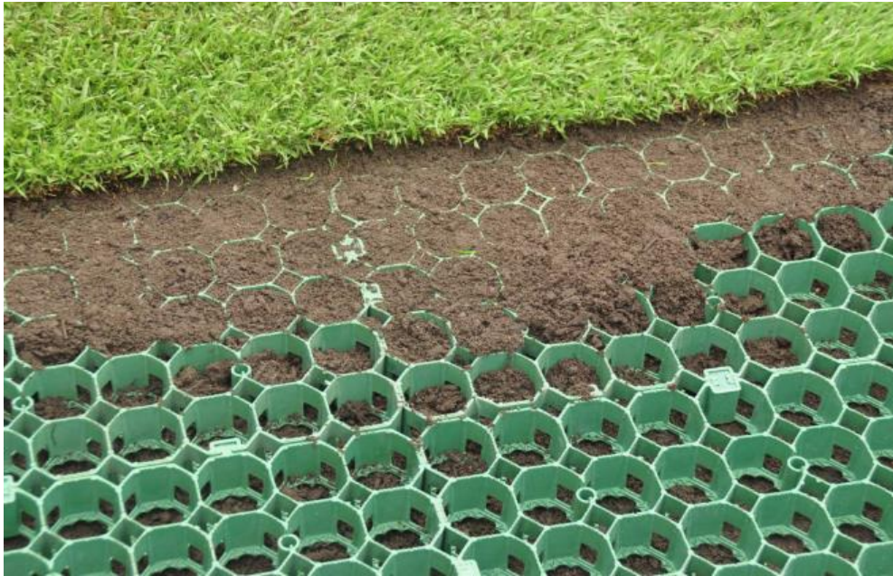
Figure 3-3 Reinforced Grass Road
