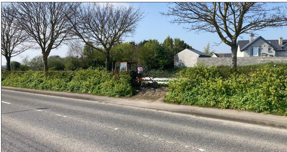
Figure 10.0 View of site from Whitestown Road, showing full use of site for market garden.
