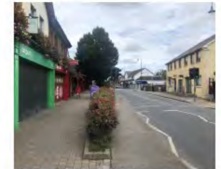
Poor positioned planting
