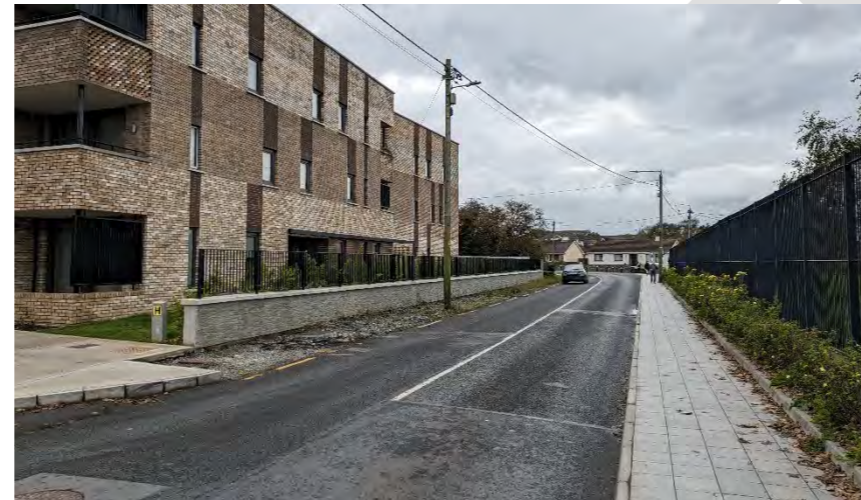
Fig. 9-1: Poor Quality Paving on Turvey Avenue
