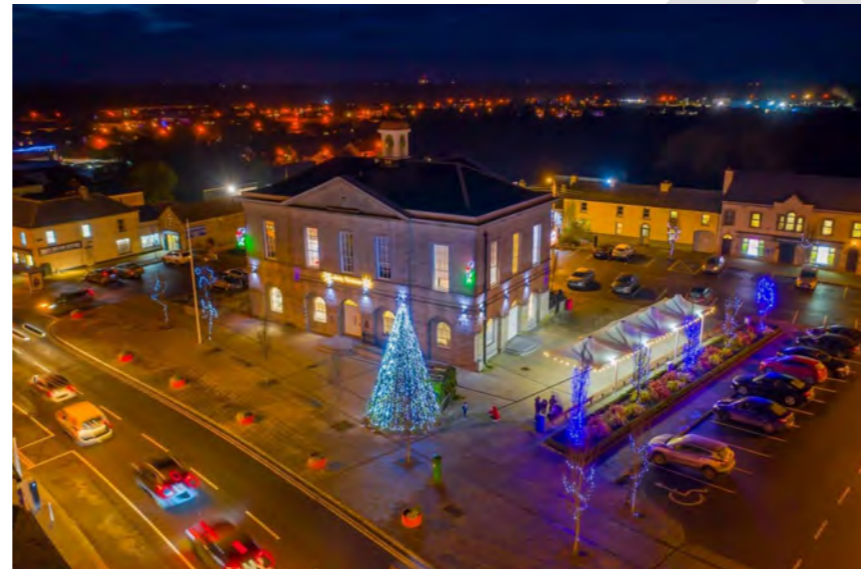
Fig. 9-1: Example of TVRS funded Public Realm Works
