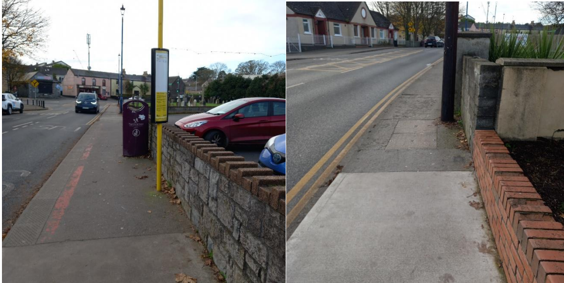
Footpath width reduced by poles, posts and litter bins.
