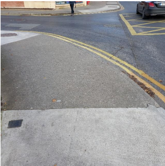
Desire lines, large radii junctions with undefined pedestrian routes close to Town Center Facilities and the lack of pavement contrast leave pedestrians, the visually impaired and mobility impaired isolated at primary crossing places.
