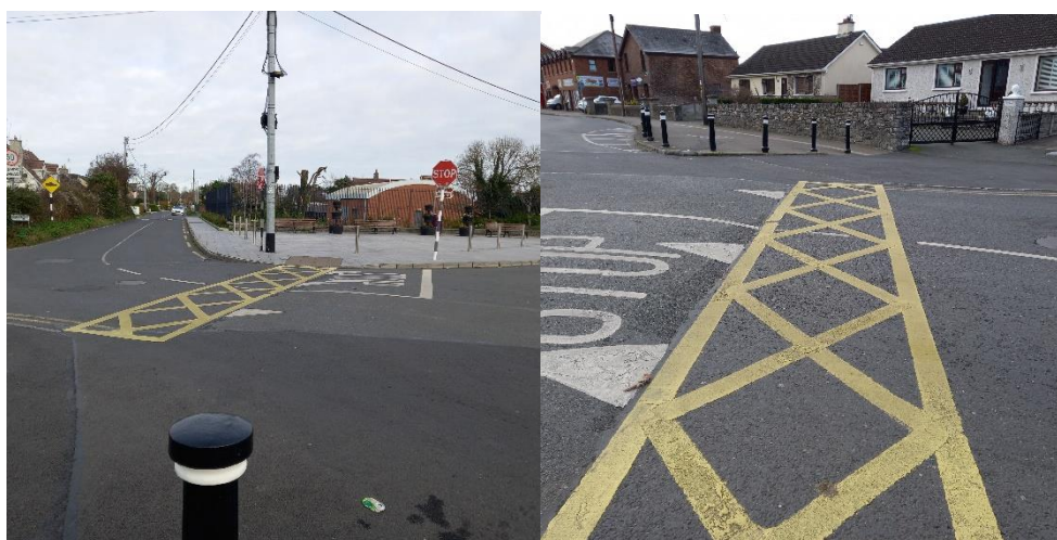
Long Uncontrolled Pedestrian Crossing Points
