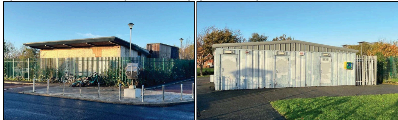
Figure 1.2: Redundant Marketing Suite and Changing Rooms/Storage Shed Structures to be Demolished
