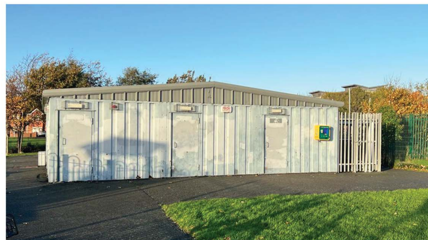
EXISTING CHANGING ROOM SHED TO BE DEMOLISHED FOLLOWING COMPLETION OF COMMUNITY CENTRE
