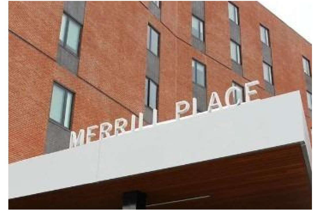
REFERENCE IMAGE - FREESTANDING ALUMINIUM LETTERING TO TOP OF CANOPY, COLOUR TO MATCH CANOPY
