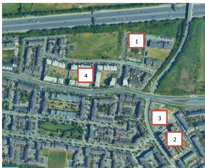
Aerial view showing nearby developments – 1: subject site, 2: Hampton Square, 3: Hampton Woods, 4: Mayeston Estate
