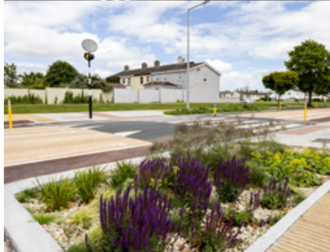
Active Travel measures in place at Brackenstown Road Swords and St Philip the Apostle School Zone
