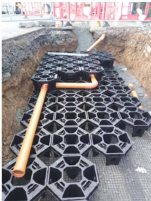
Tree pit under construction
