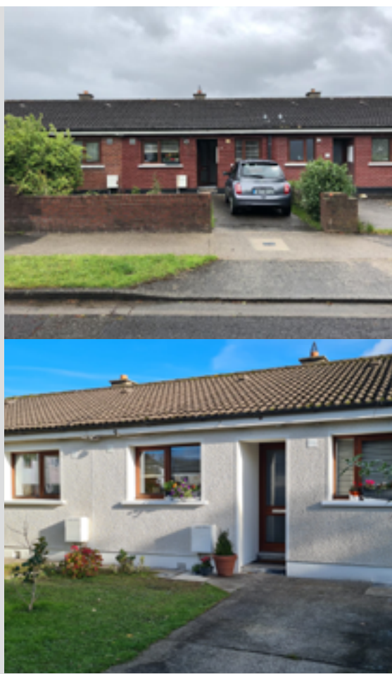
Greenridge court before and after Energy Efficiency upgrades
