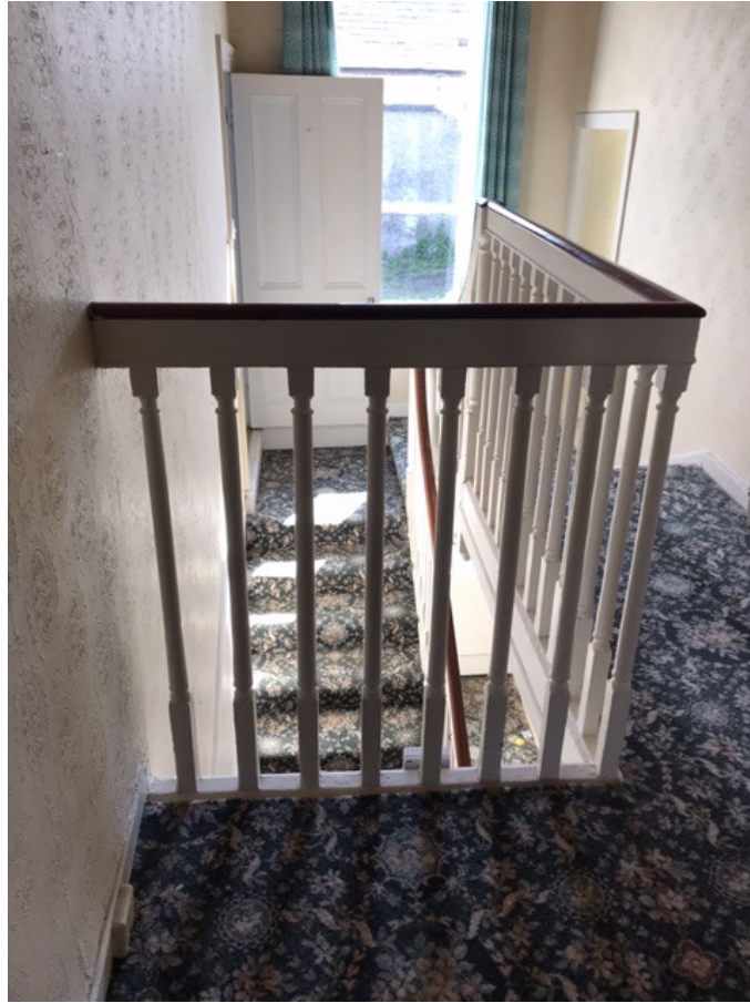
Stairs Timber Balustrade
