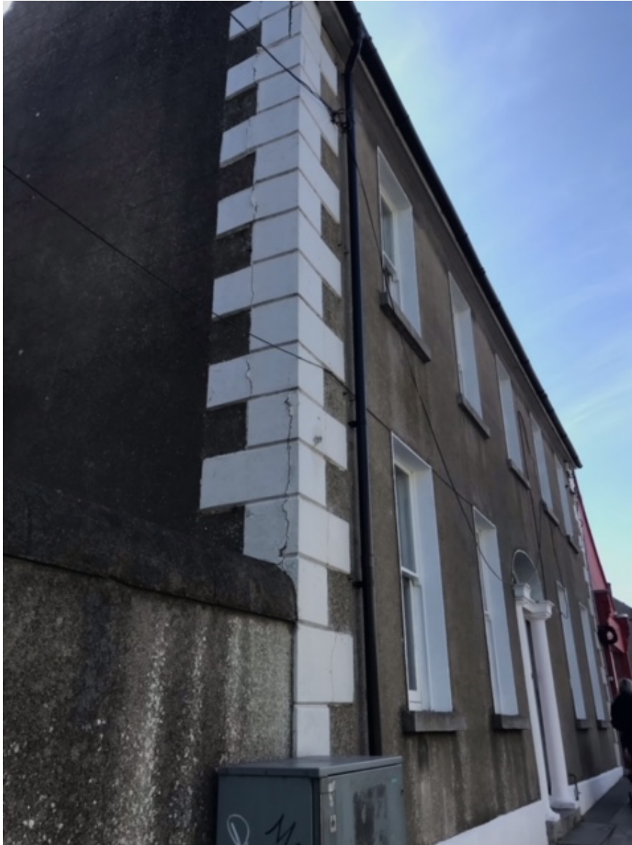
Northwest Corner of 2-4 Dublin Street
