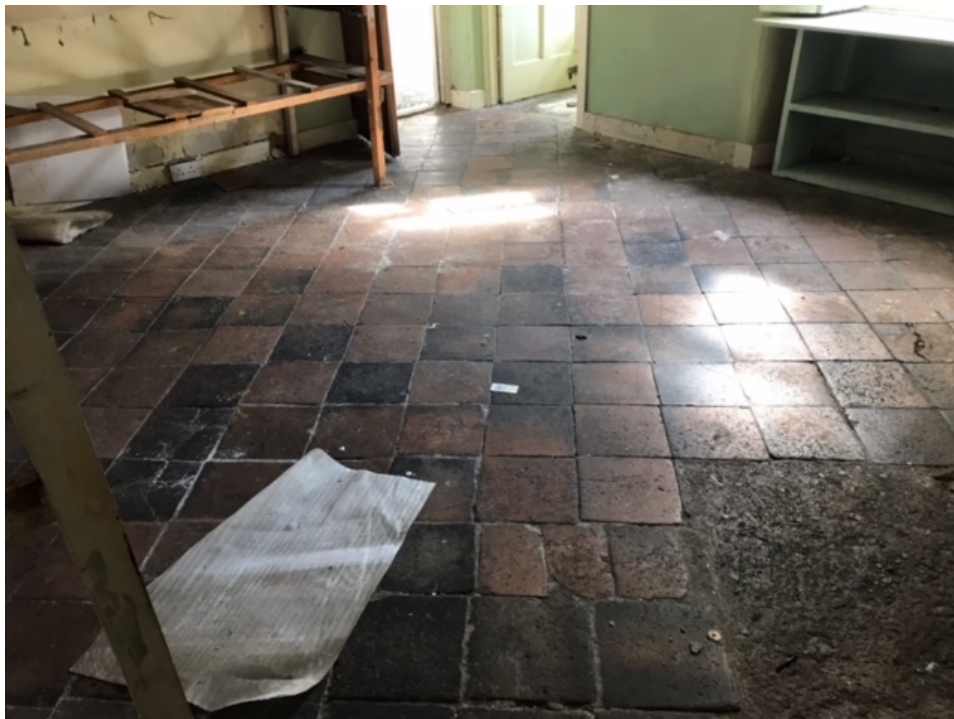
Ground Floor Tiled Floor
