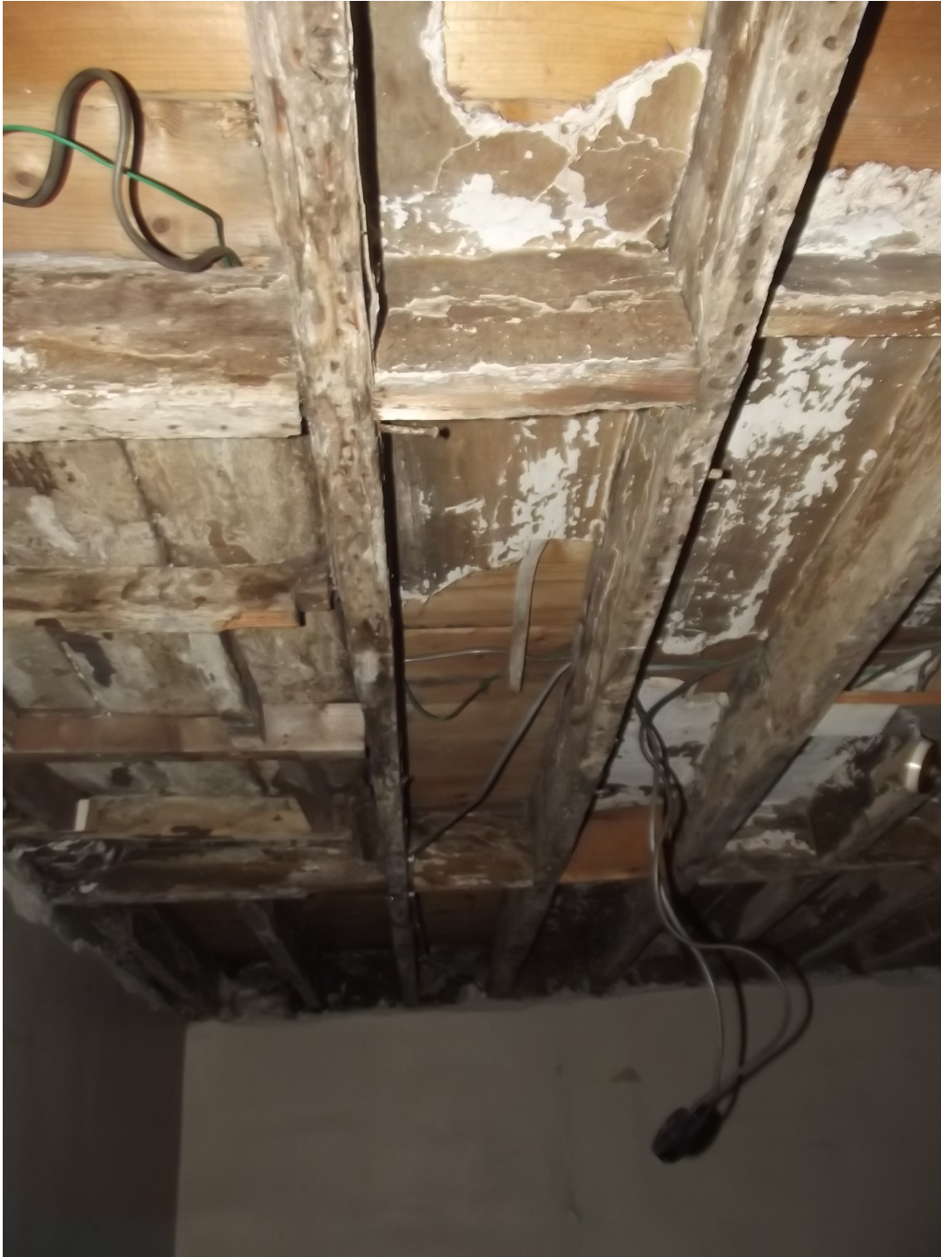
Figure 3. Underside of first floor, southeast corner, showing early limewash to joists.
