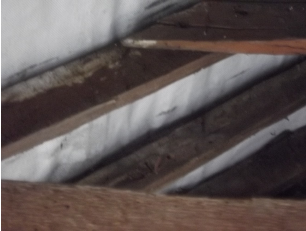
Figure 4. Original rafters, with mortar marks to top edge (top LH corner)
