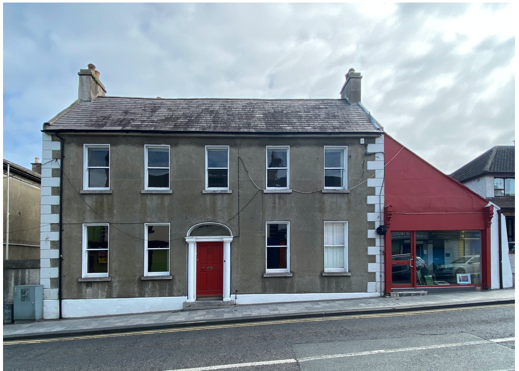
2-4 Dublin Street, Front Façade
