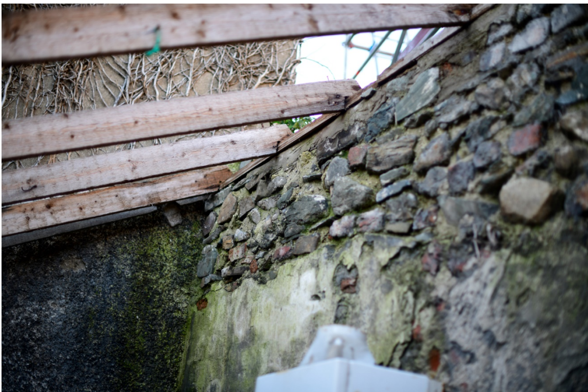
Plate 2. Stone Masonry exterior to the site.
