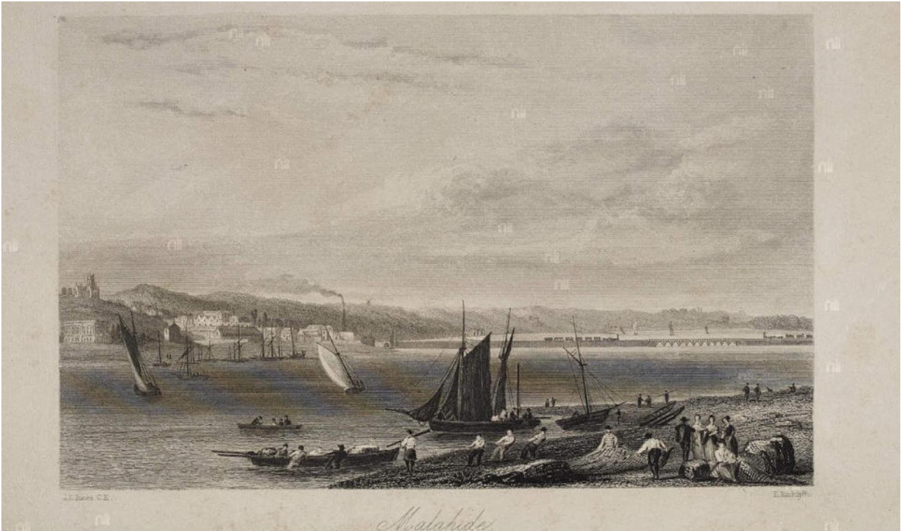
Malahide in 1844, note the new railway line spanning the estuary
