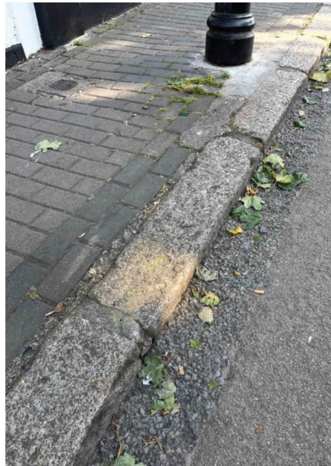
Fig. 79: New Street Existing Kerbing
