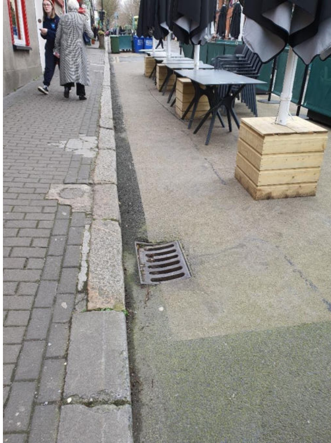
Image 5: Existing gullies present along New Street.
