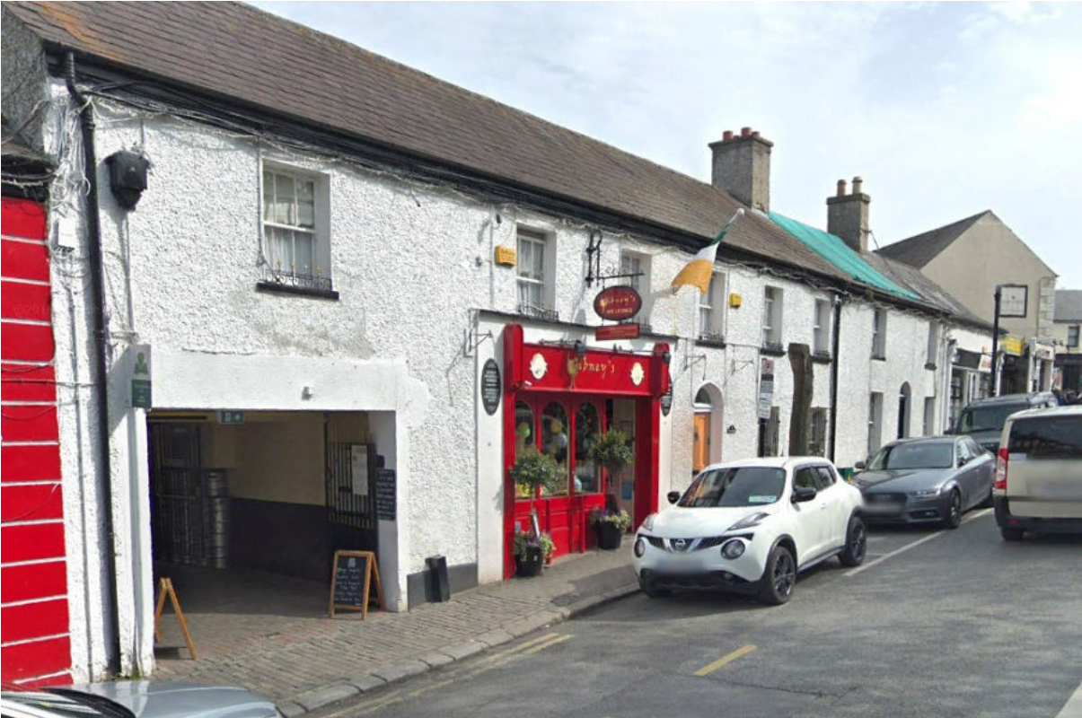
19th century house on the eastern side of New Street
