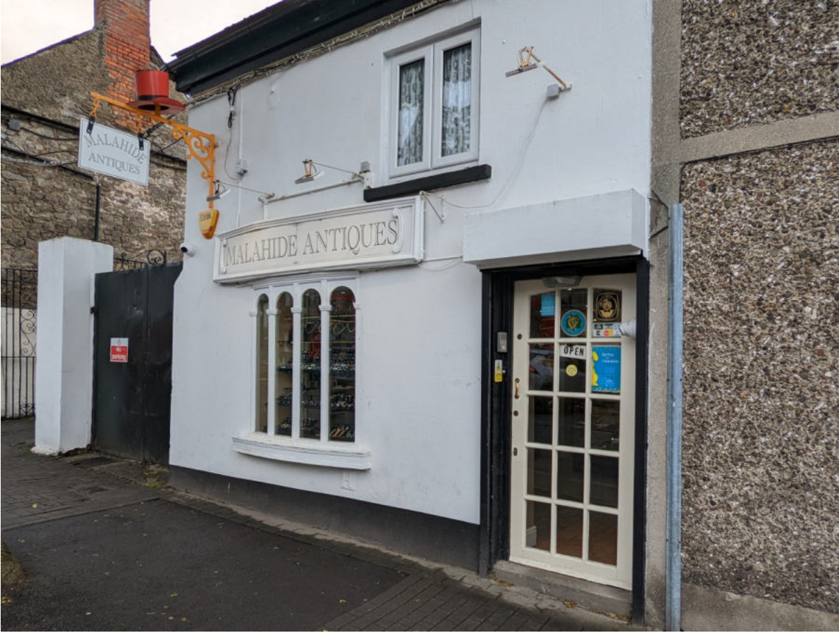
The northern of two historic storefronts with bowed windows
