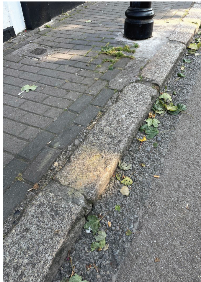
Fig. 79: New Street Existing Kerbing
