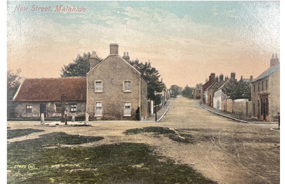
Fig. 39: (View B) New Street - Image taken from Strand Street.
