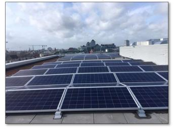
The energy balance for this mixed-use scheme means that a decentralised heat pump scheme with supplementary photovoltaic would be the most practical option for meeting the renewable energy requirements.
