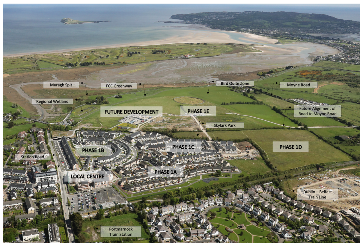
Figure 7: Drone Image showing the extent of development within the Portmarnock landbank by Quintain to date.
