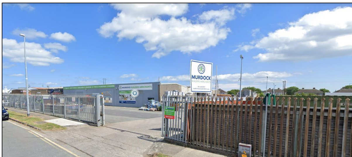
Figure 5.0 Street view image of the existing access from Kilbarrack Parade to our clients' lands.
