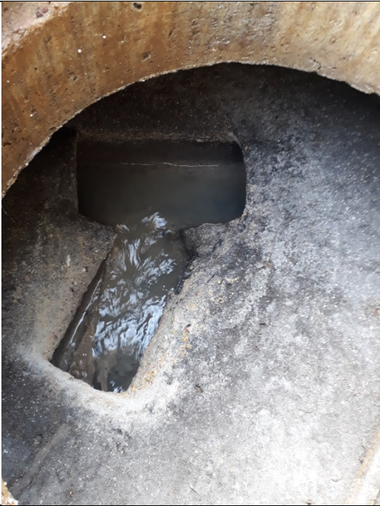
The SWO at the inlet manhole
