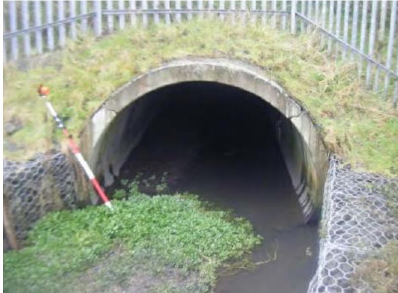
Figure 5-2 Culvert under the M1 on the LAP Lands
