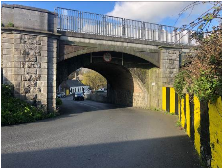
Bridge Height Restriction 3.2m from Quay Street to Seapoint
