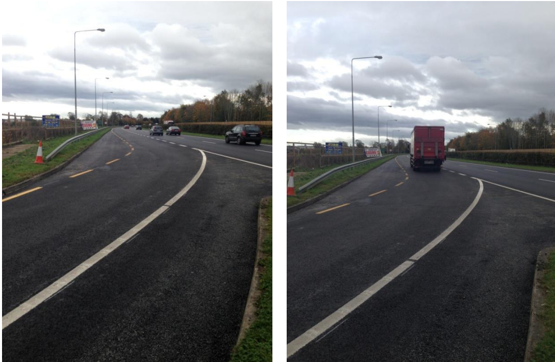
Figure AppC-7-2 - Existing parallel merge at Parslickstown Junction (hatching now in place)
