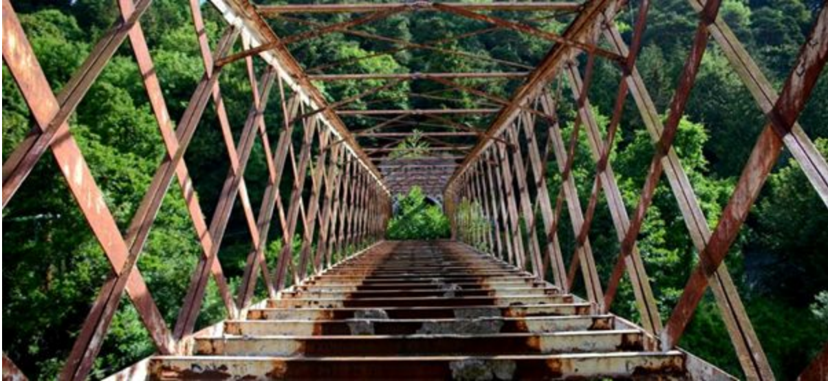
Photo taken on the inside of the structure.
