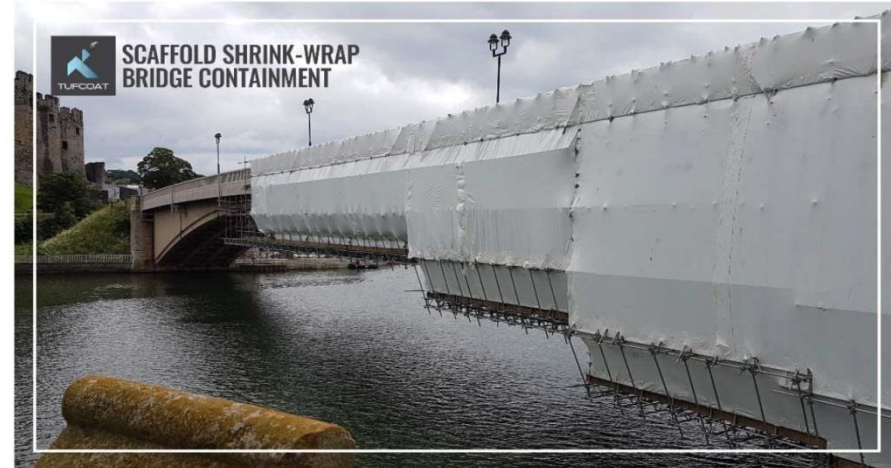
Samples of shrink wrapped scaffolded bridges
