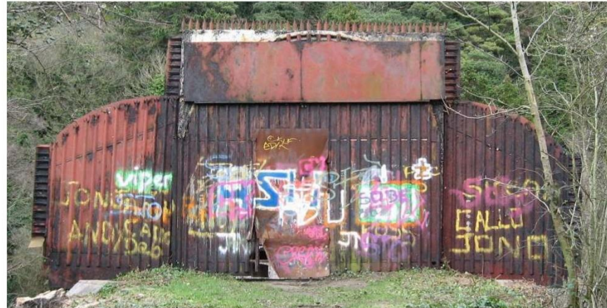
Existing gate at south bank - external view
