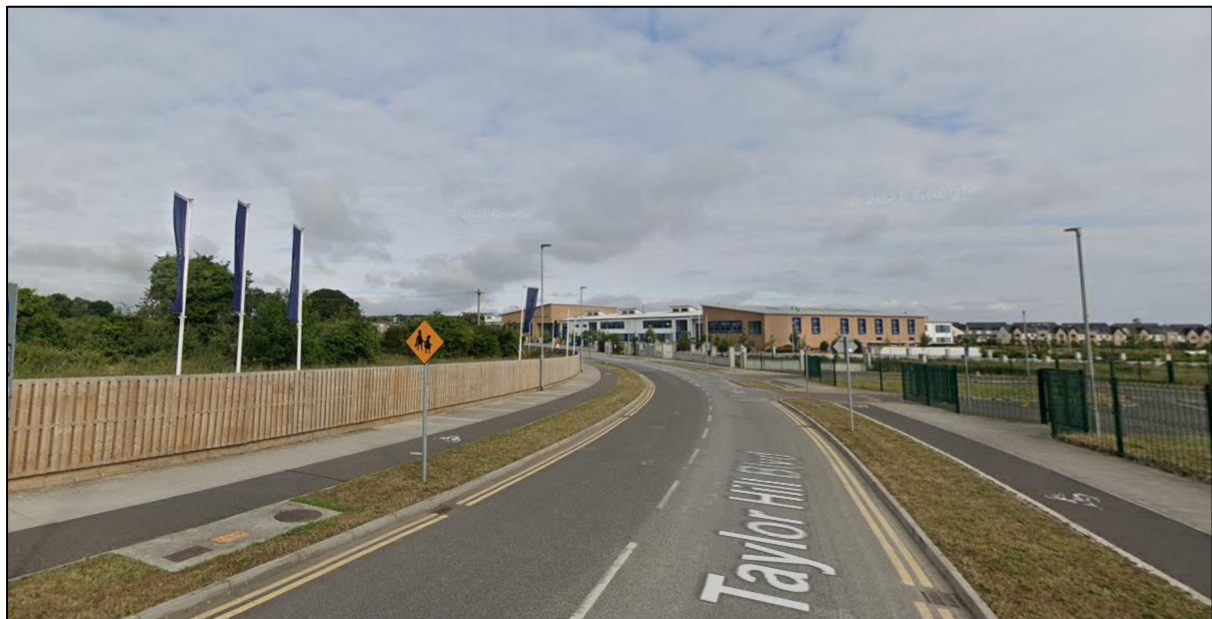
Figure 9.0 Street view image showing the completed section of the Taylor Hill Boulevard Road
