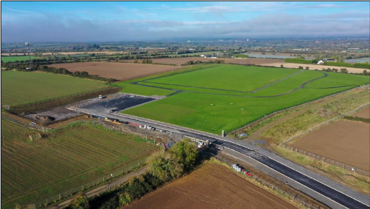
Figure 32.0 Drone image showing the completed Class 1 Pitch at Balbriggan north-west.
