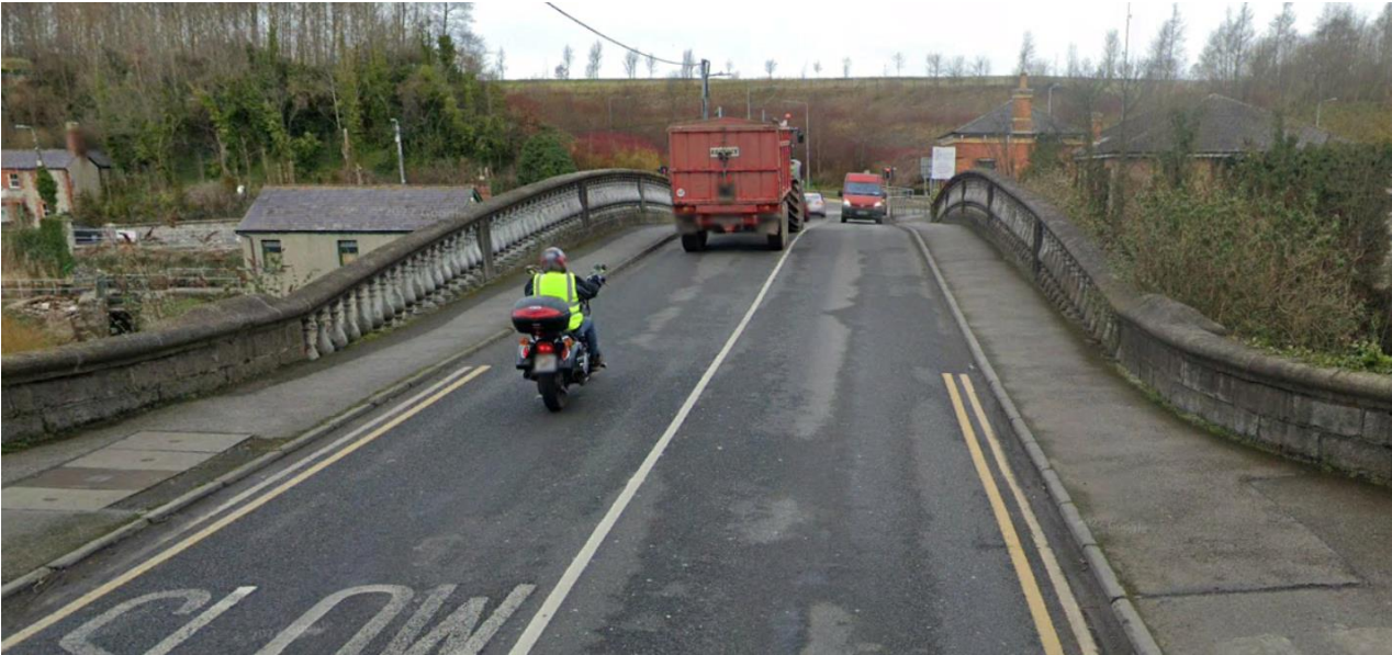
Figure 2.5 Photo of Lucan Bridge (looking northwards toward signalised junction)
