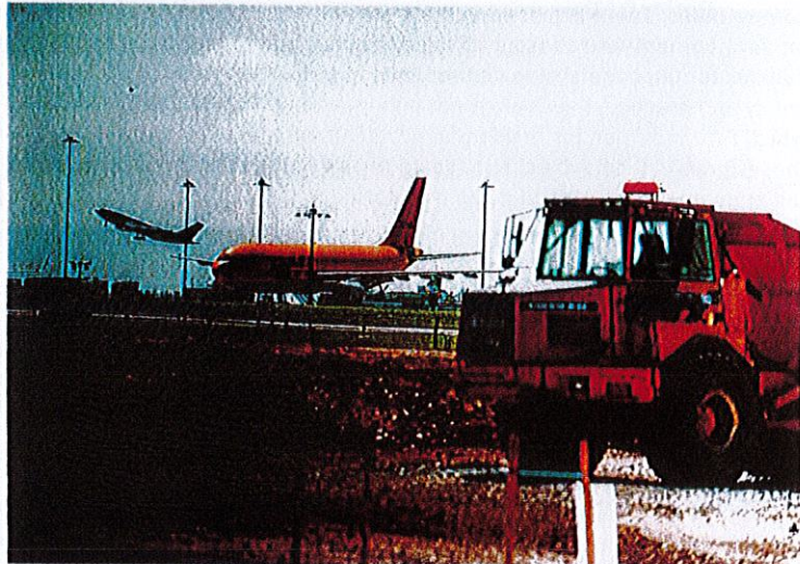
Business as usual during the construction of Dublin airport's north runway
