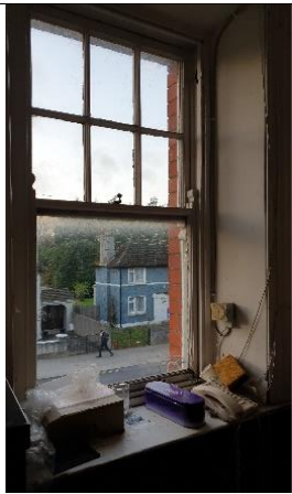
Figure 5 6 over 1 single glazed sliding sash / painted soft wood
