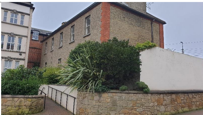
Figure 3 Change in level at rear of building with soil and plant built up against east and north walls, possible source water ingress.
