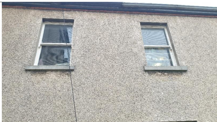
Figure 5 General view of east elevation
