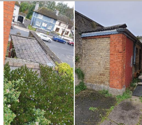
Figure 6 View of mon-pitched roof to out house
