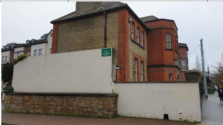
Figure 1 North elevation with buff coloured brick to main walls in an English Cross or Dutch Bond with alternating rows of header and stretcher.
