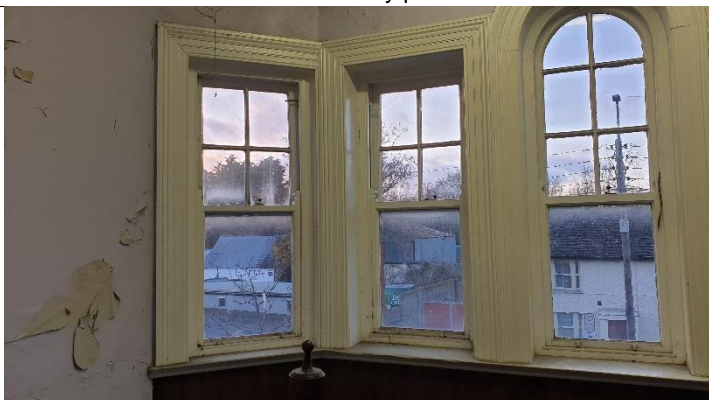
Figure 3 Two of 5 windows to LHS
