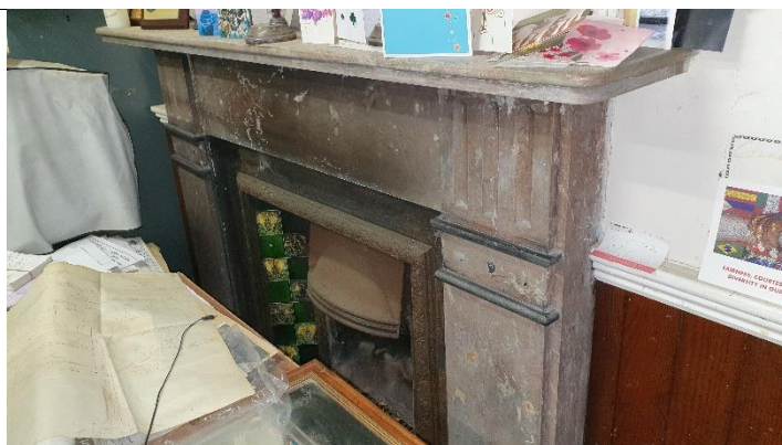
Figure 6 -marble fireplace with cast iron insert Some missing decorative stones at top of LHS and RHS pilaster -
