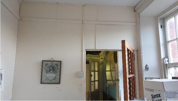
Figure 1 2500mm stud work with plaster board ceiling within main space
