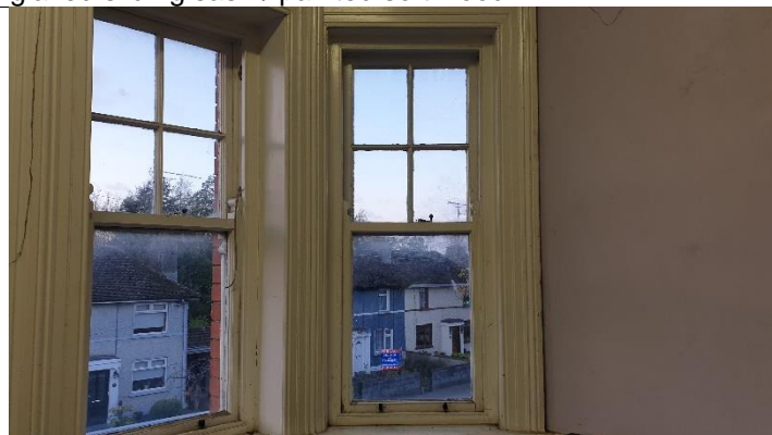
Figure 4 Two of 5 windows to RHS
