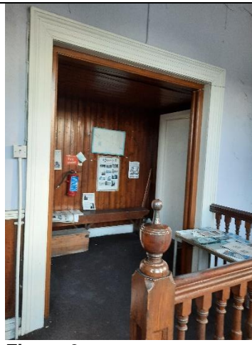
Figure 6 Original profiled painted soft wood architraves to opening to lobby
