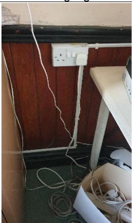
Figure 7 lime plaster walls to upper section with 900mm high stained softwood wainscoting
