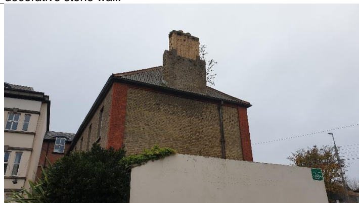
Figure 4 Wall to out-house appears to be in-situ concrete in sections. Cracks in cementitious render
