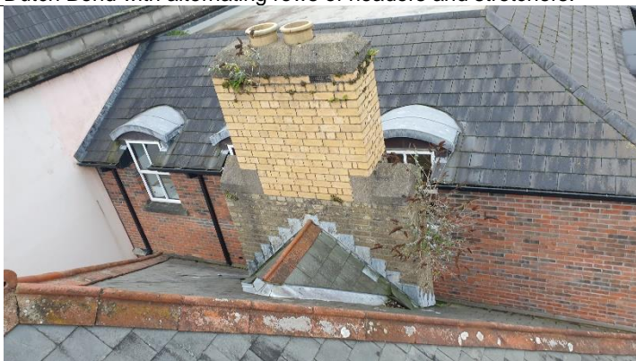
Figure 5 Neighbouring building overlooking south facade
