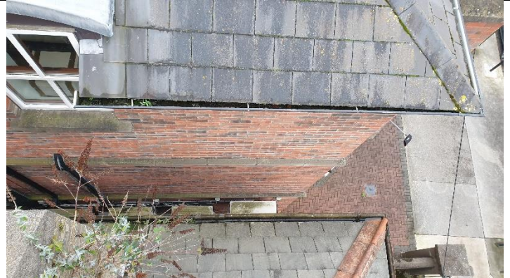
Figure 6 View of gap between south elevation and neighbouring building
