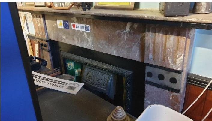
Figure 5 - marble fireplace to north wall with cast iron insert
