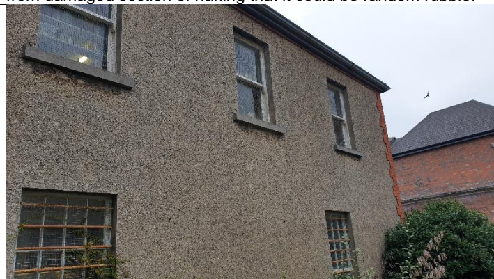
Figure 6 General view of east elevation – towards north-east
