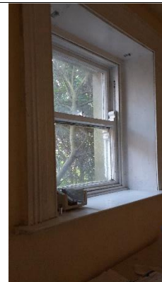
Figure 8 One over one Original painted softwood window with surrounds
