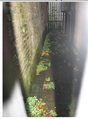
Figure 8 Low level view of gap between structures
