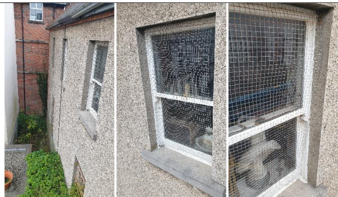
Figure 7 Wire mesh in front of external windows
