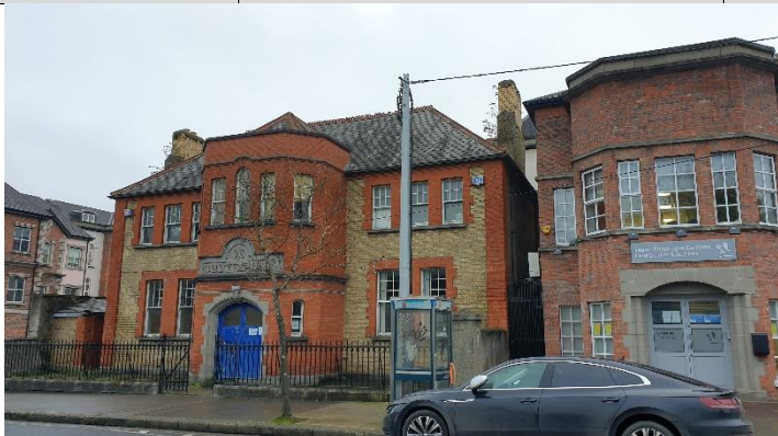
Figure 1 West elevation showing south elevation at gap next to neighbouring modern construction.
