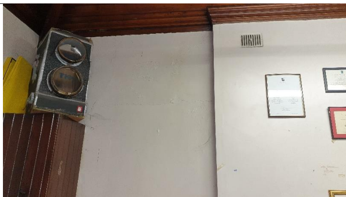
Figure 8 Damage to plaster at south gable wall due to water ingress from gutters
