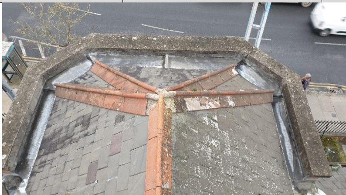
Figure 1- Roof outcrop above stairs with hexagonal bay and hips
