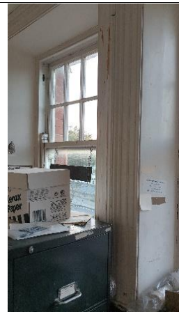
Figure 6 6 over 1 single glazed sliding sash / painted soft wood
