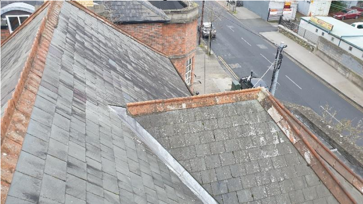
Figure 5 Roof outcrop above stairs with hexagonal bay and hips
