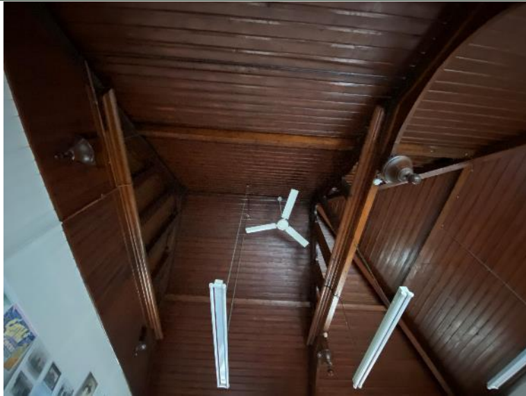
A5. First floor ceiling of main building.
