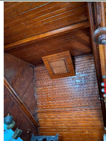
A4. First floor ceiling of main building.
