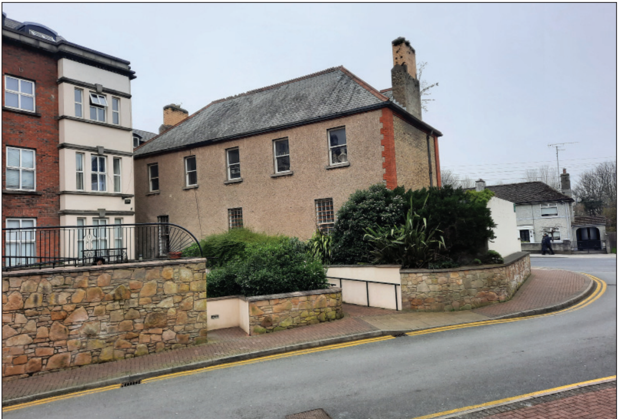
Plate 2 - Rear of Carnegie Library (CH007), facing southwest
