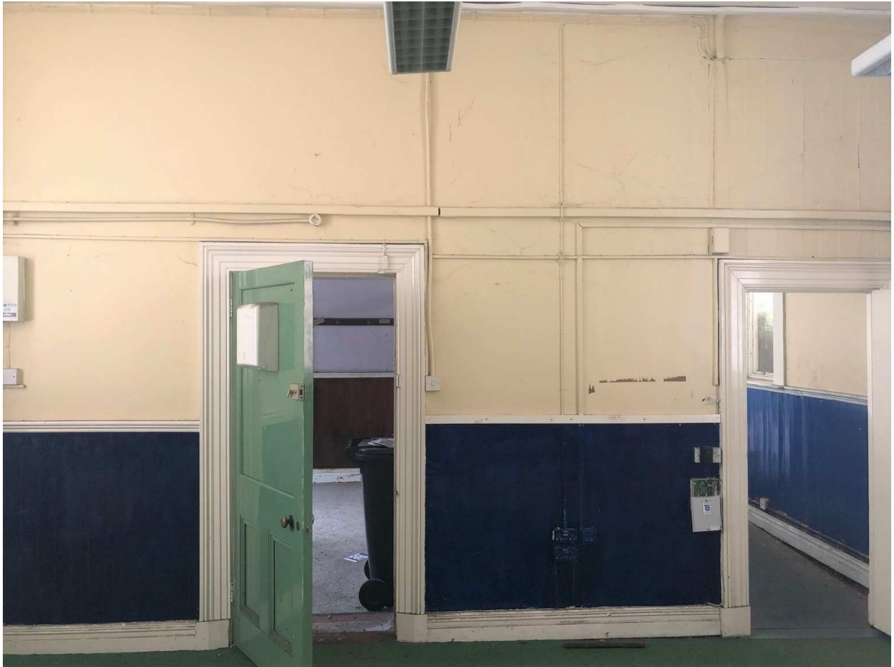
Fig 13: Room G-01 – Room North Elevation
