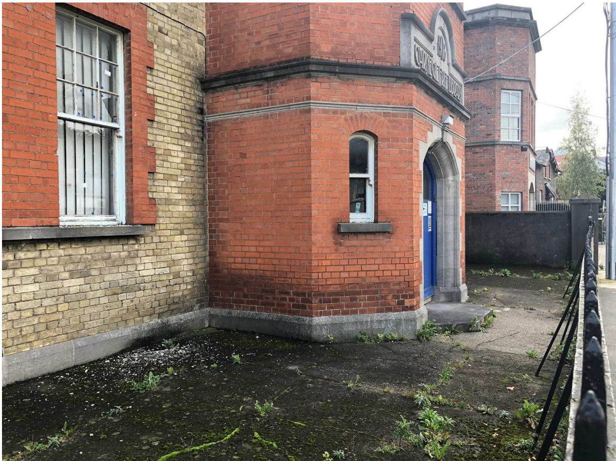
Fig 6: Entrance – North Street
