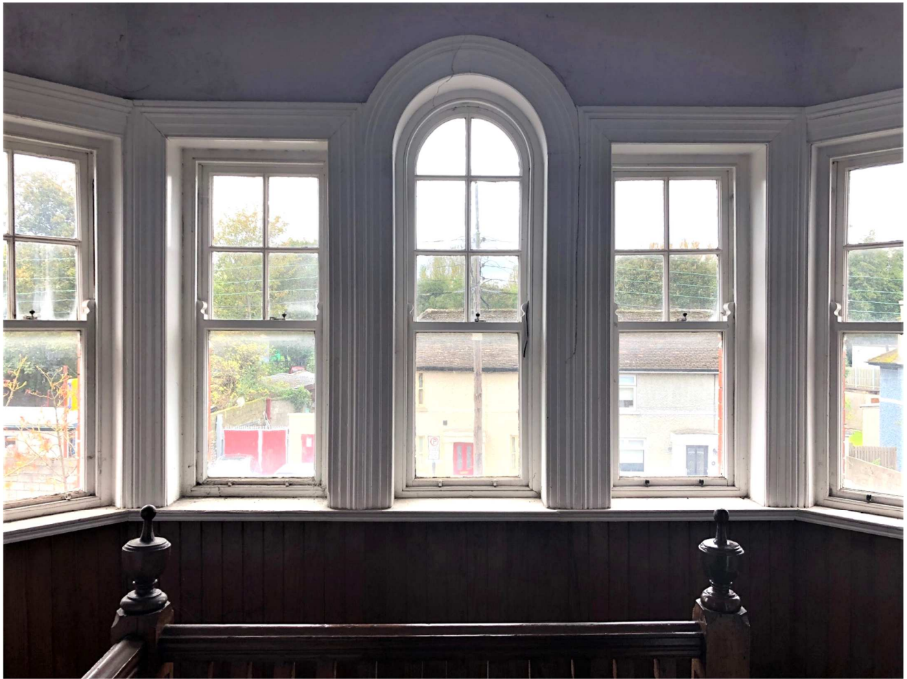
Fig 16: Room F-04 – Room West Elevation
