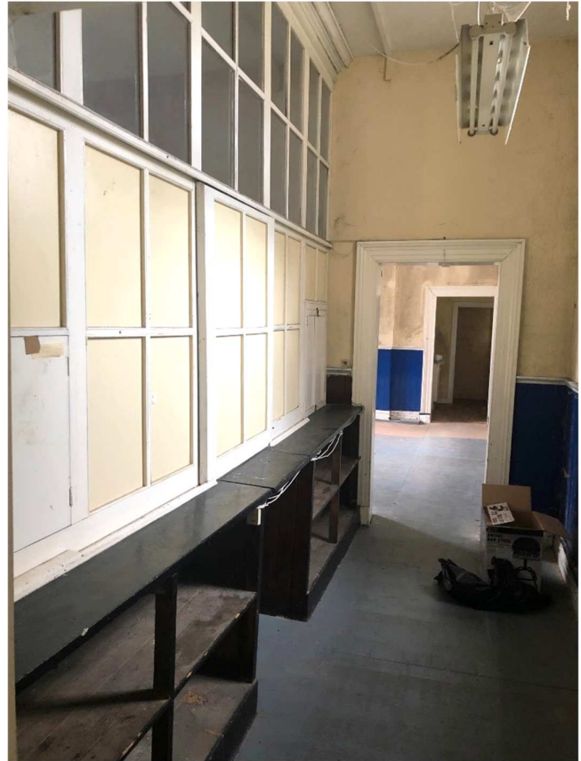
Fig 11: Room G-03 – Room North Elevation
