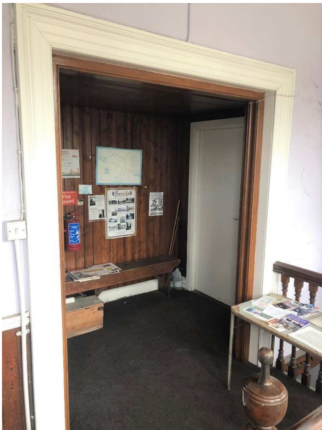
Fig 14: View of Room F-03
