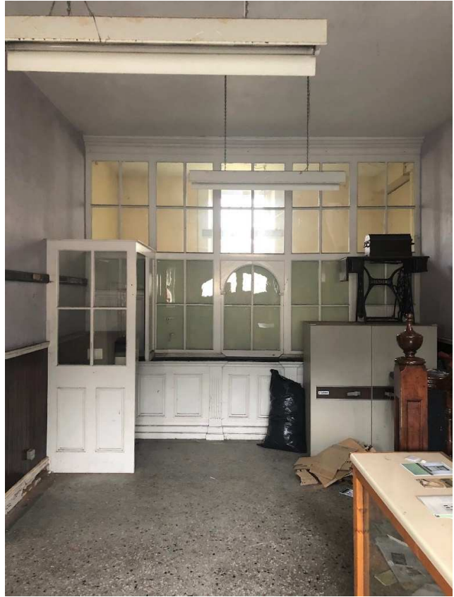
Fig 8: Room G-02 – Screen / Counter
