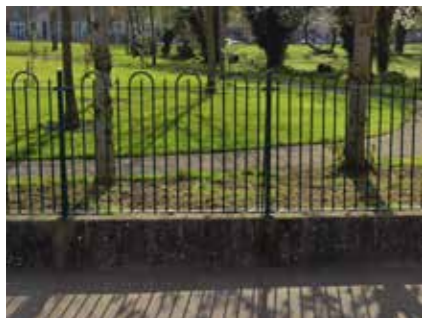
Concrete Plinth and Steel Railing Fence
