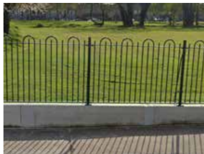
Concrete Plinth and Steel Railing Fence
