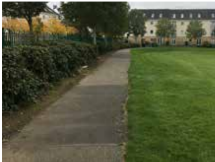
Internal Asphalt Footpath
