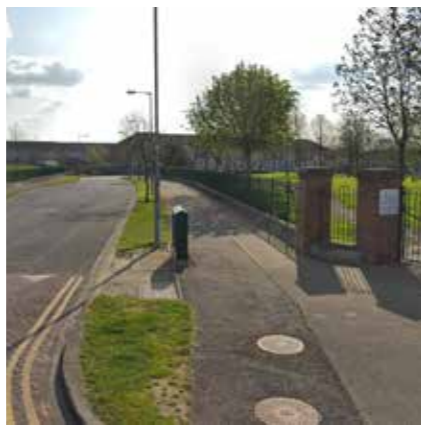
External Asphalt Footpath - Lanesborough Rd
