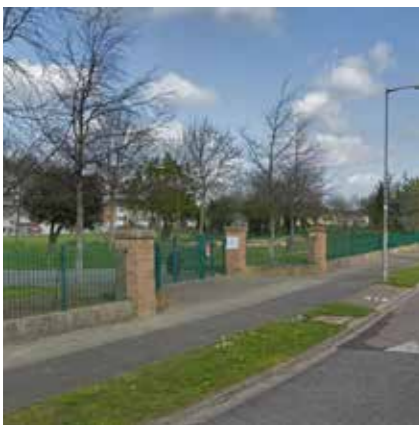
External Asphalt Footpath - Lanesborough Rd
