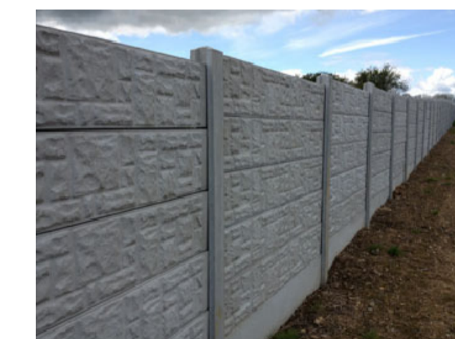
2m high Concrete panel wall
