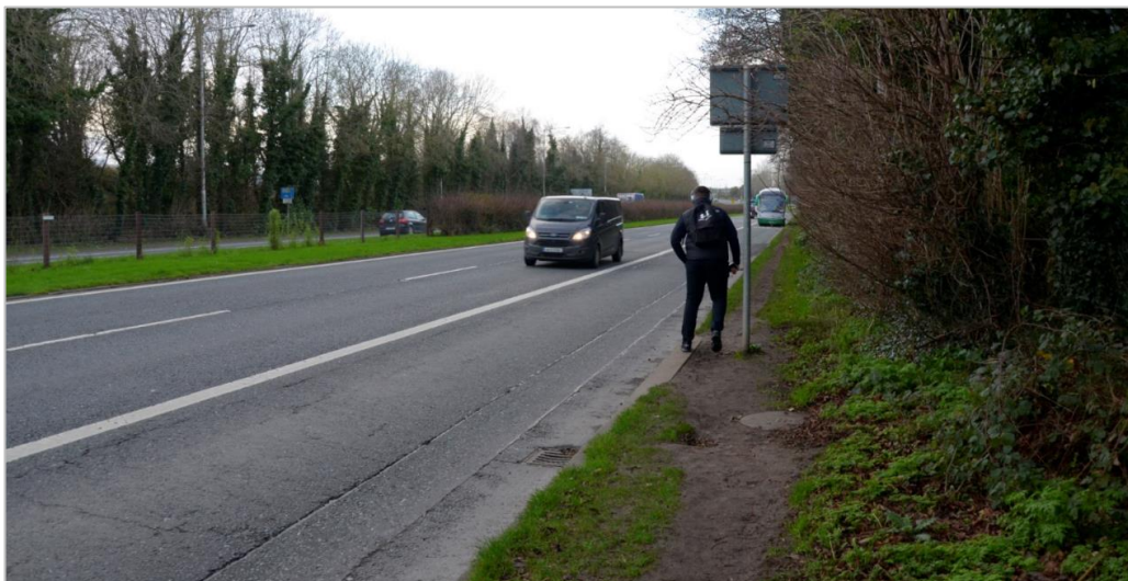
Figure 3.1: Lack of Pedestrian Infrastructure along key Desire Lines
