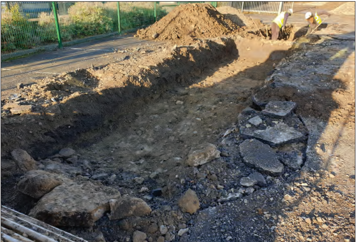
Plate 10 - Trench 4, looking northwest
