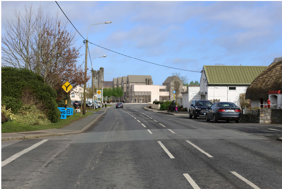
View Approaching the Site
