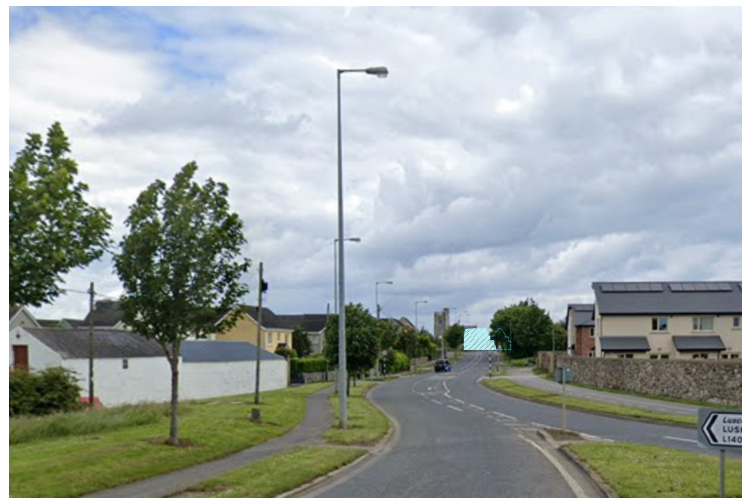
View as Exiting Southern Roundabout – Ecclesiastical Site / Proposed Building Visible
