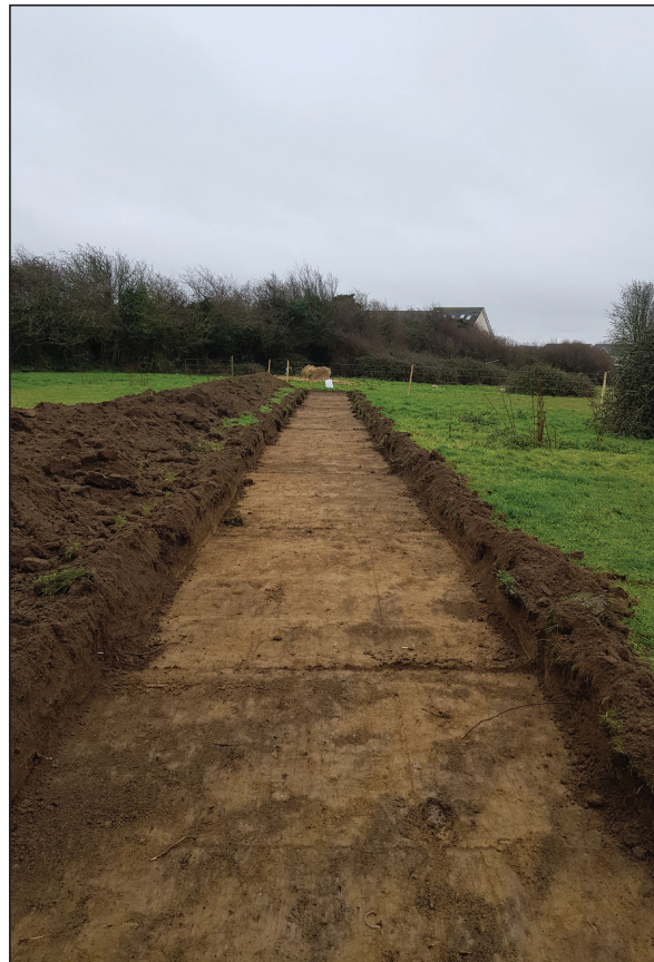
Plate 2 - Trench 1 overview looking SE
