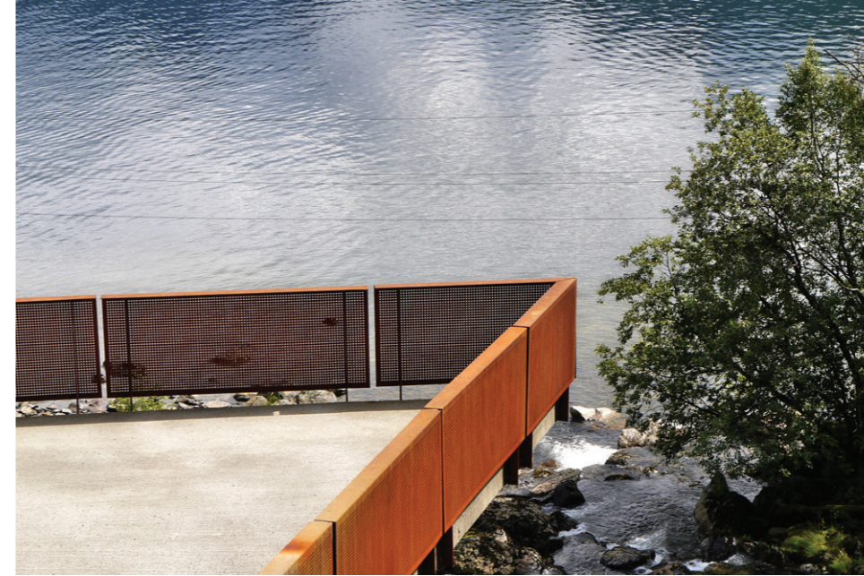
Materiality of upstand - corten and walking surface - corten or concrete strips to allow for permeability
