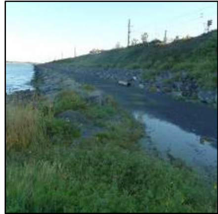
Plate 8. Existing hardcore maintenance access track on embankment to South of Viaduct.
