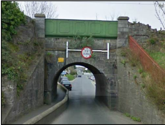
Plate 7. Bissets Bridge (view from east side).
