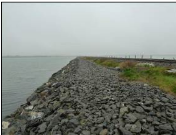
Plate 9. Stone Embankment to North of Viaduct looking North.
