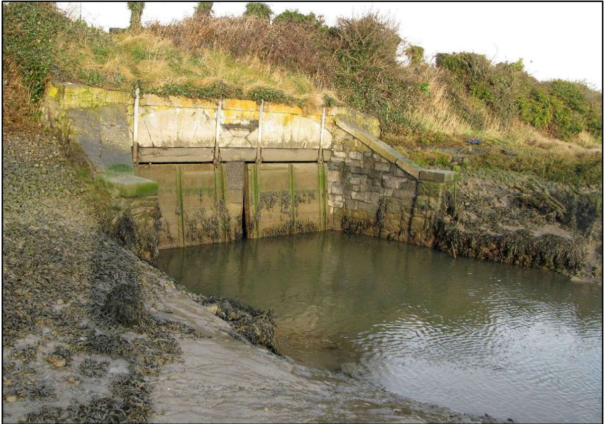
Plate 3: View of the tidal flaps on the River Pill outlet beneath the railway embankment viewed from the Malahide Estuary side.
