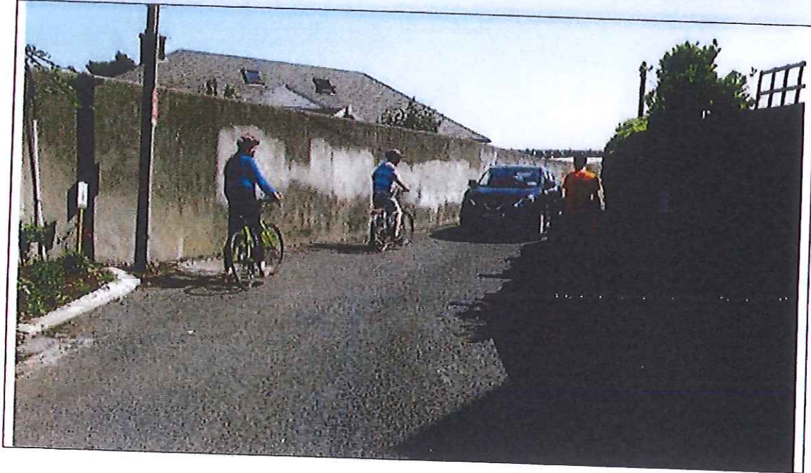
Photograph 4: Hazardous lines of sight into oncoming vehicular traffic for users at O'Hanlon's lane northern end
