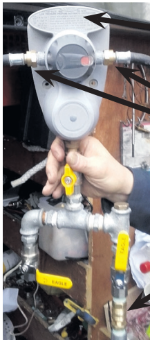
Photograph 9: Low pressure regulator
