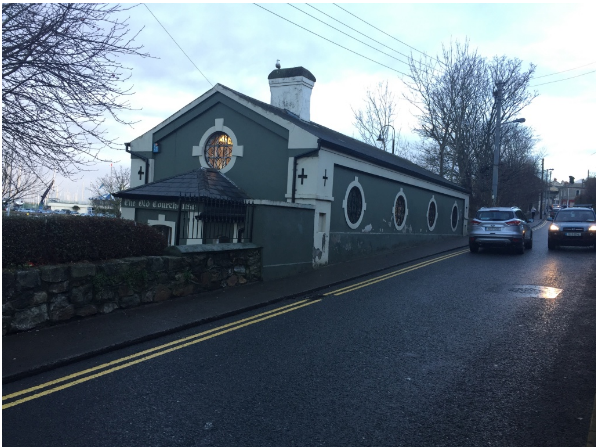
Plate 2. Exterior view of Southern side of building. The circular windows at either end of the elevation are currently blocked up and it is proposed that these windows are opened up to provide natural light to the interior of the building. All existing windows within these opes will be repaired and re-decorated.
