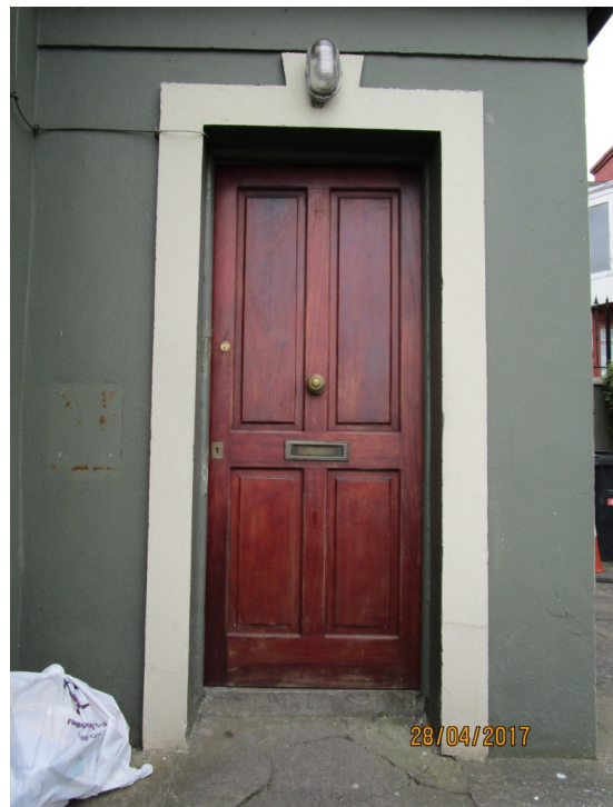
Plate 5. Entrance door on Porch.
