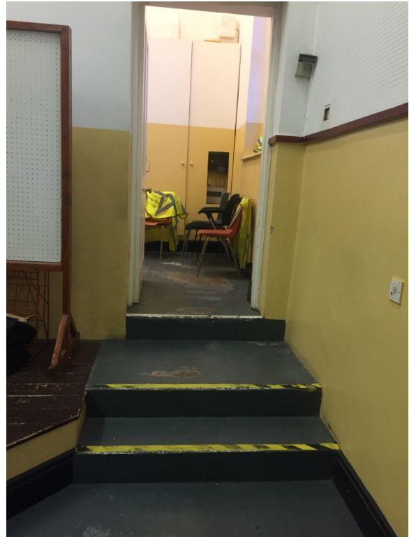
Plate 11. Photo illustrating difference in level between main hall and small western room. A ramp is proposed as part of the works to facilitate disabled access between these two rooms.
