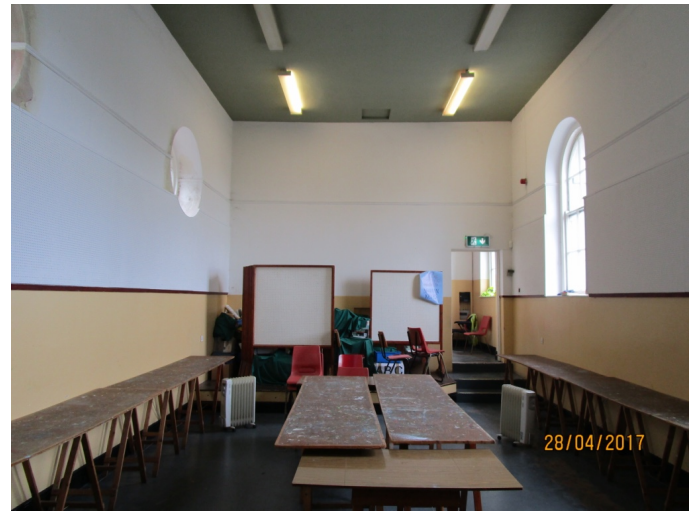
Plate 9. Interior of main hall looking West. It is proposed to remove the existing peg board from the walls and return the walls to a simple plain plaster finish. New pendant lighting is also proposed within the space. The current raised stage at the end of the hall will also be removed as part of the works. This stage does not appear to be original and was probably used when the building was used as a courthouse.
