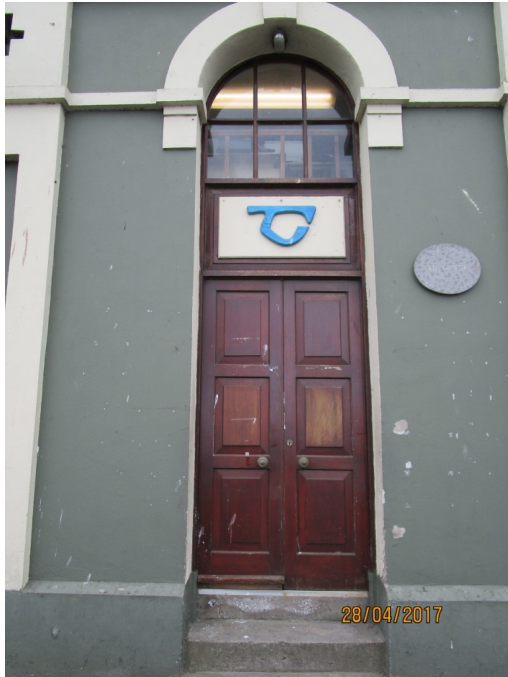
Plate 6. Door on North elevation.
