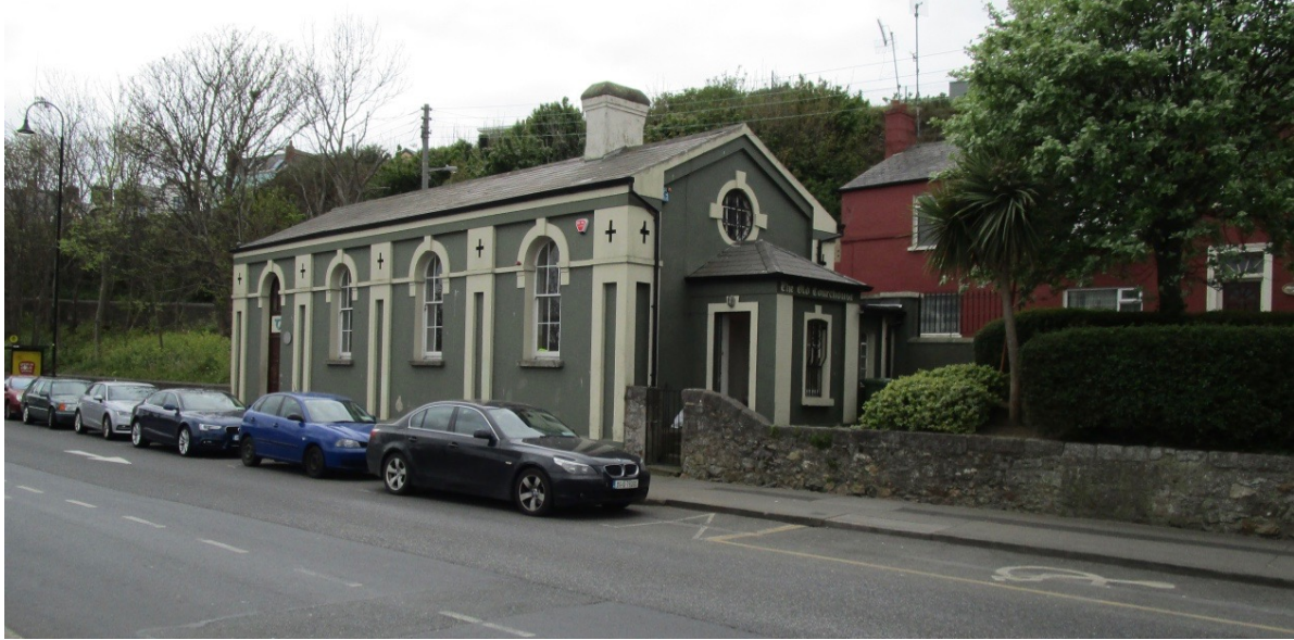
Plate 1. Exterior view of Northern side of building.
