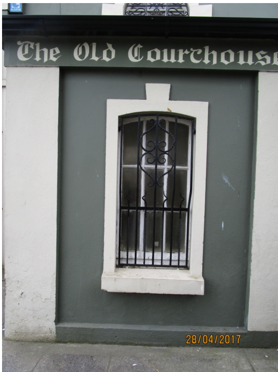
Plate 4 Porch window on west elevation.
