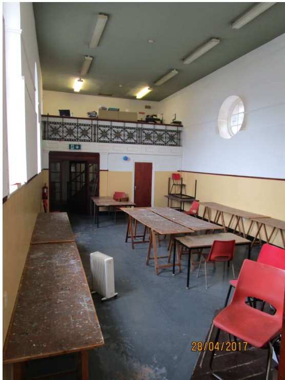
Plate 8. Interior of main hall looking East to mezzanine floor. A small tea station and store is proposed under this balcony, which will involve the addition of 2no. new doors to match the existing four panel doors within the building.
