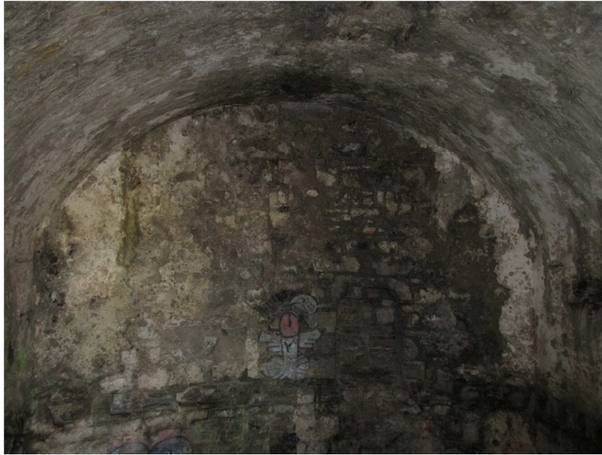
Plate 47: Interior of the Martello tower, first floor
