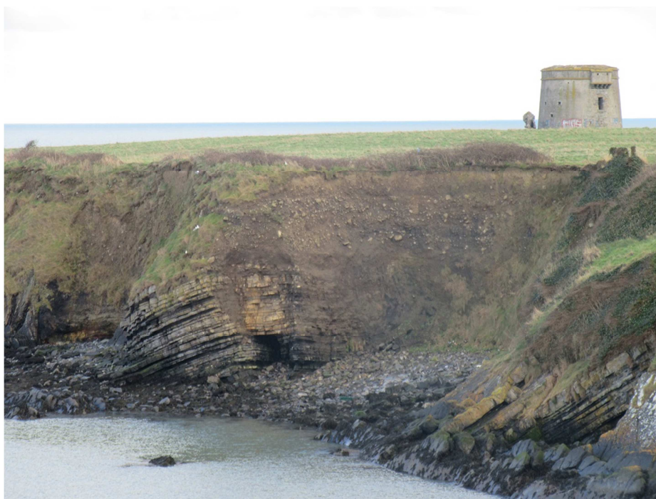
Plate 35: View of erosion along the northern perimeter of Drumanagh
