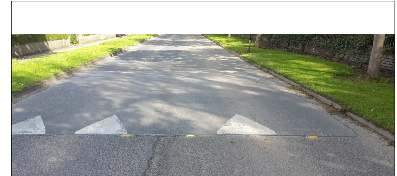
TYPICAL TRAFFIC CALMING RAMP
