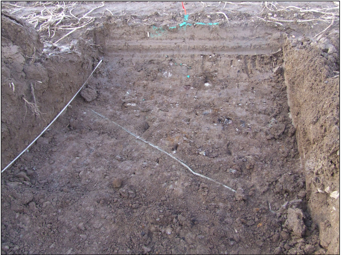
Plate 9 Detail of disused modern copper pipe at W end of BT9 (Field 12)
