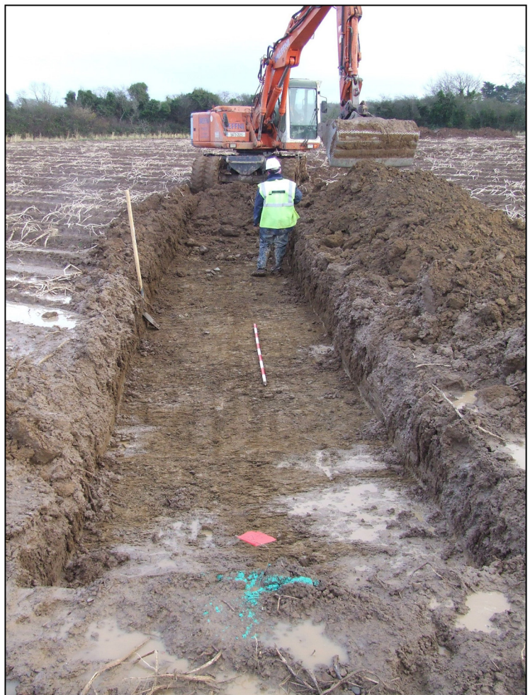
Plate 2 View NE of excavation of BT8 (Field 12)
