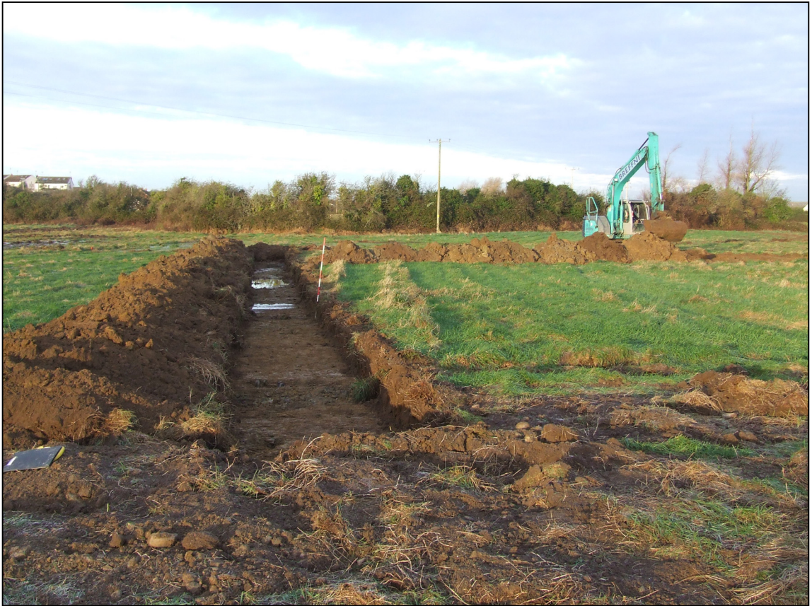
Plate 1 View W of backfilling of BT17 and BT16 (Field 17)
