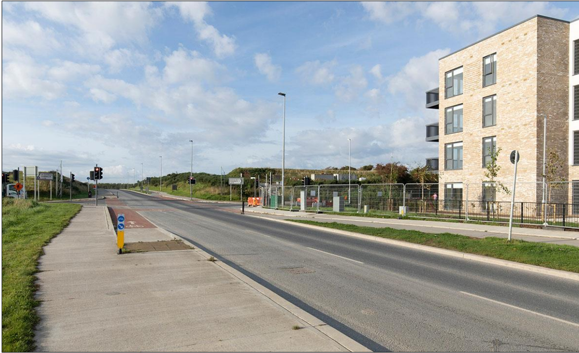
Figure 2.2: South-east corner of the site with residential development permitted under Fingal County Council Reg. Ref. F20A/0510 / An Bord Pleanála Case Reference PLo6F.311447 (as amended By Fingal County Council Reg. Ref. F22A/0686) on the right-hand side of the frame
