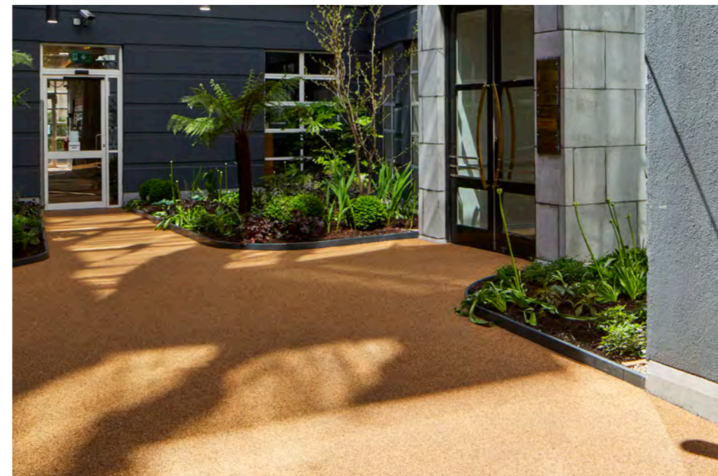
Resinbound gravel to the Communal Open Space
