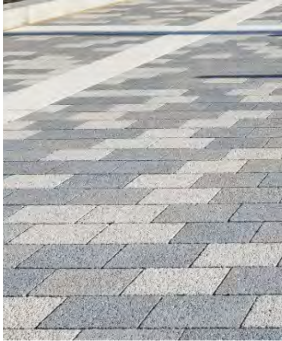
Block Paving to the environs of apartment buildings.
