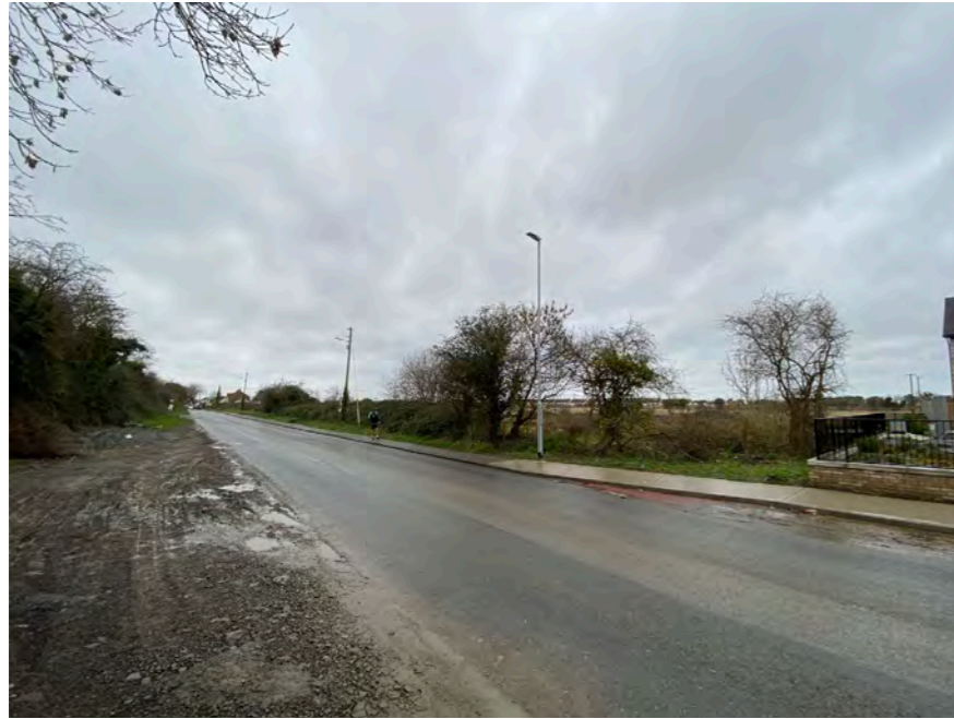
View of south east corner of site from New Road.
