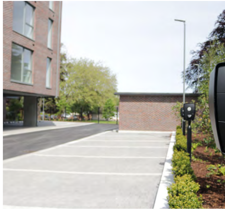
Permeable block paving to parking spaces.
