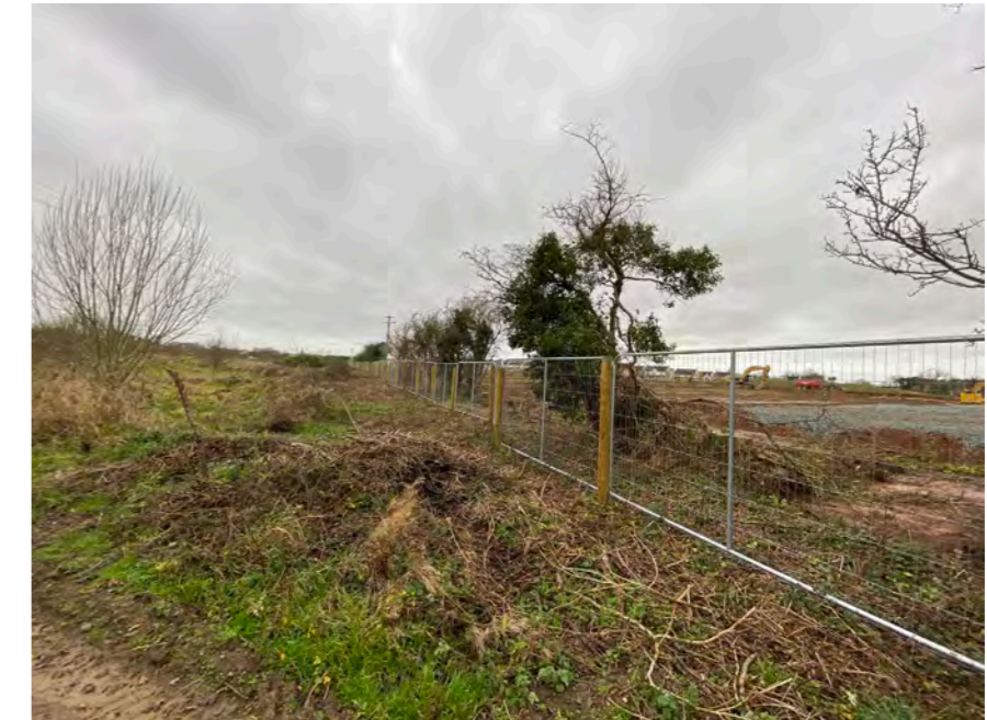
View along northern site boundary looking west. Temporary construction site fencing for Ballymastone development visible on RHS.
