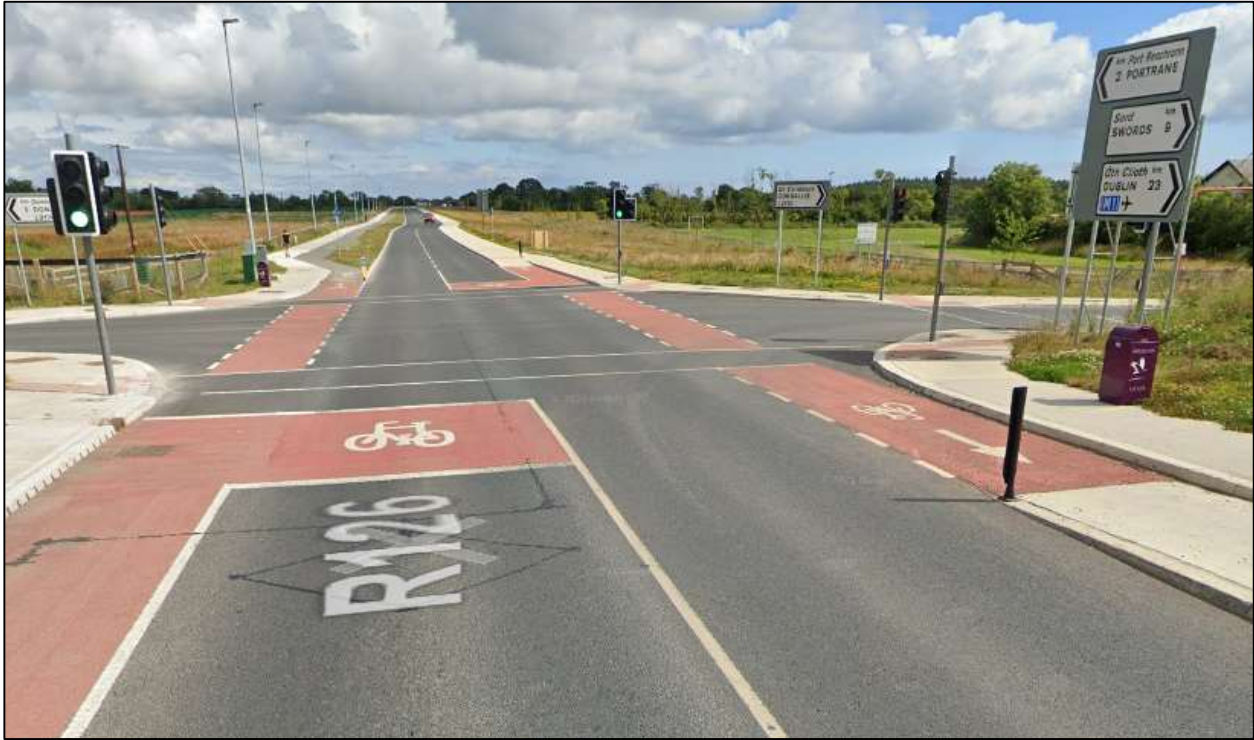
Figure 18 | Existing Cycle facilities currently exist at the intersection of Donabate Distributer Road and New Road (source Google July 2021).
