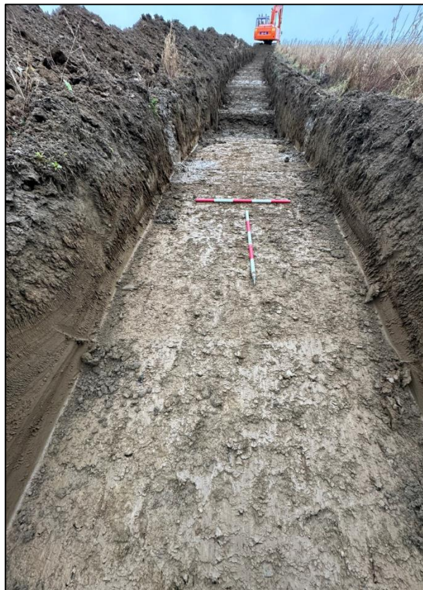
Plate 17 Test trench 8 view looking west upslope
